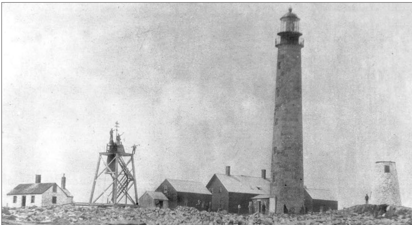
When reporting on Mount Desert Rock, Matinicus Rock, and Saddleback Ledge in Maine in 1843, I.W.P. Lewis wrote, "These four places are lone rocks, standing several miles from shore. There is nothing but the naked barren rock & the lighthouses, for the eye to rest upon. In storms the sea break furiously over the buildings & the keepers & their families are in danger of being swept away. Nothing can well be imagined more desolate & uncomfortable than such situation. All supplies of stores & fuel are necessarily obtained from the mainland during the summer season as these rocks are inaccessible during the fall & winter" This ca. 1859 photo shows the third tower (and the shorter tower it replaced) on Boon Island. Photo courtesy of USCG Historian's Office.
