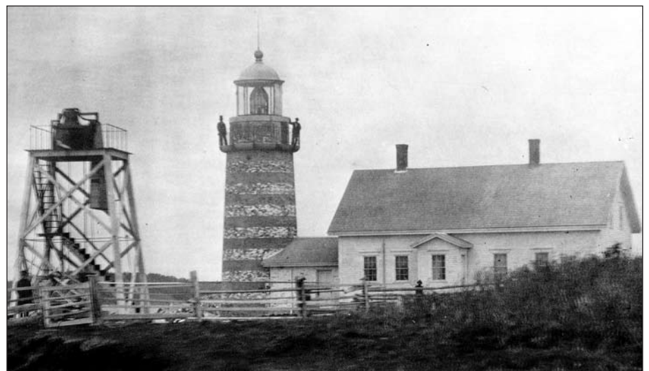
According to the 1819 salary survey, the station at West Quoddy or Passamaquoddy "has the advantage of Wood, but is situated in a cold part of the County where provisions are always high." This ca. 1859 photo shows the new tower recently constructed at West Quoddy Head. Photo courtesy of National Archives.
