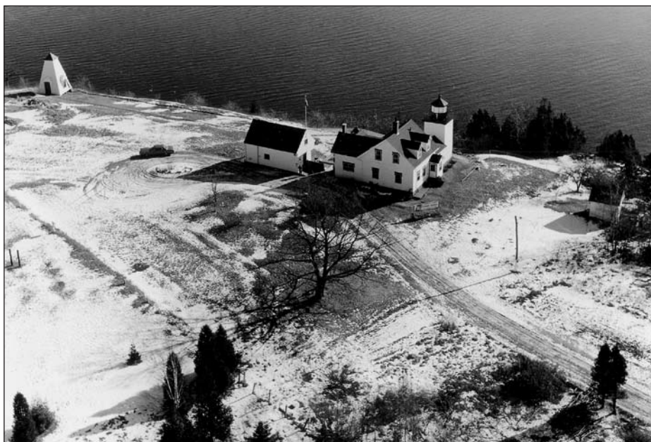
Fort Point Light Station, Maine had good soil and acreage for a garden. Fog bell tower at left, garage (old barn) next to dwelling. Photo courtesy of the U. S. Coast Guard.
