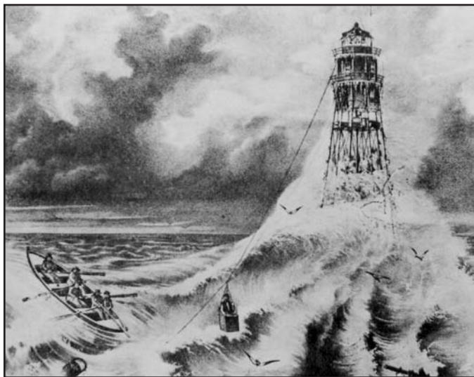
Landing supplies at Minots Ledge. The line from the lighthouse was secured to a large boulder on the seabed and may have helped cause the destruction of the tower.
