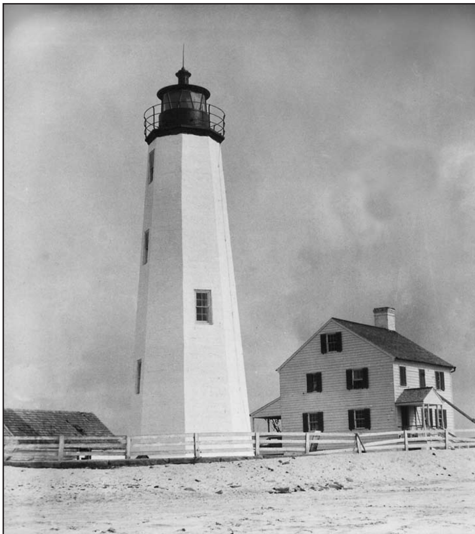
New Point Comfort Light Station in the 19th century. Note the lantern astragals (bars holding glass) are trapezoid shaped and the lantern vent is the old style. National Archives photo.
