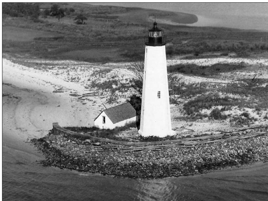
New Point Comfort on June 27, 1928 before the area around the tower broke away from the larger island. Note the lens still in the lantern room. The dwelling has been removed but the barn remains. Photo courtesy of the Coast Guard.
